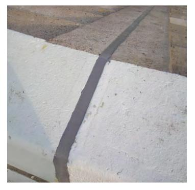
THIOKOL® sealants have been developed for aggressive chemical and fuel containment areas. These chemical resistant sealant systems offer long-term protection from intermittent and continuous exposures to organic and inorganic acids, caustics, solvents and fuels.
